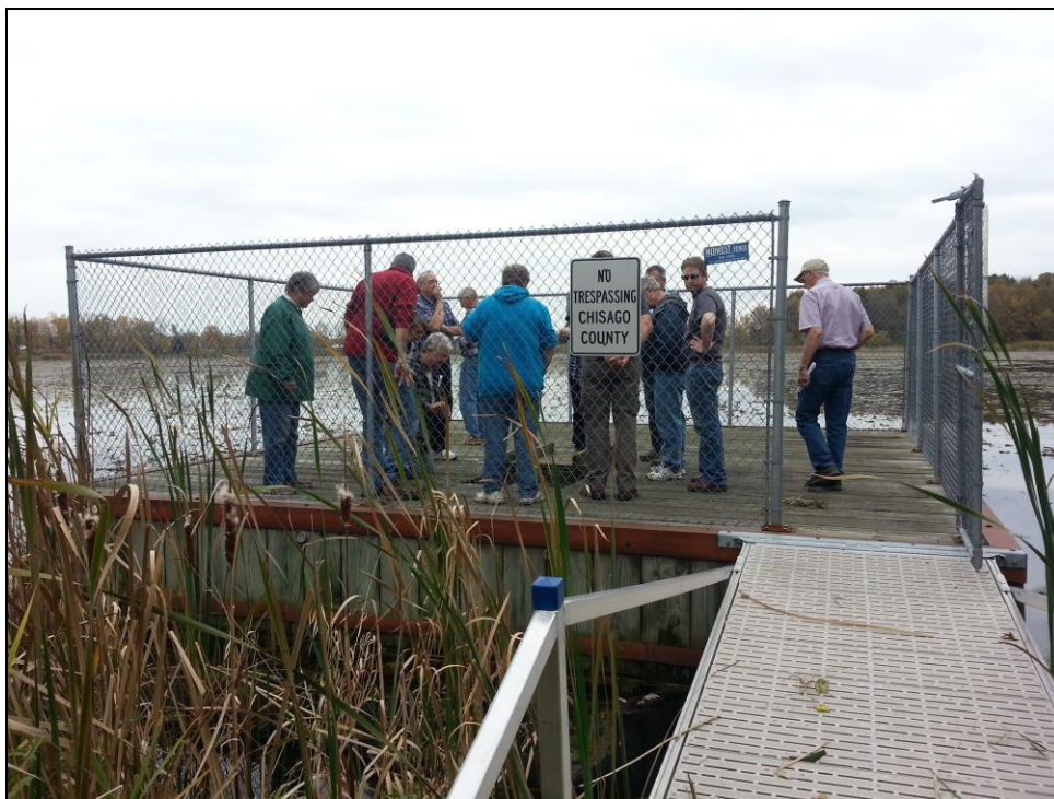
Photo: Ramp leading to weir structure.
