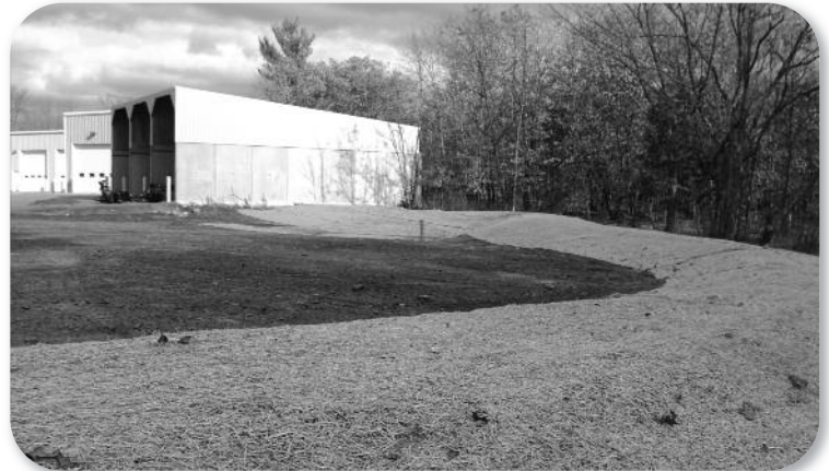
Taylors Falls Public Works Facility gully stabilization project (Gully Inventory)
