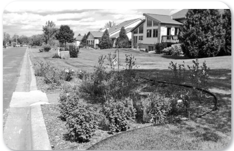
Curbside rain garden in Lindstrom (Urban Subwatershed Retrofit Assessment)
